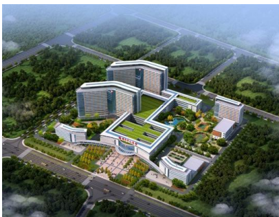
Suizhou Central Hospital
