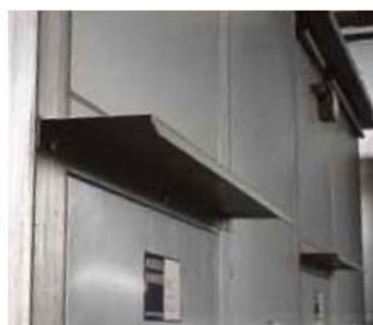
Overhanging eaves above the inspection door
